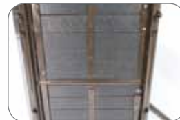
Indestructible rubber panels in alley gate
