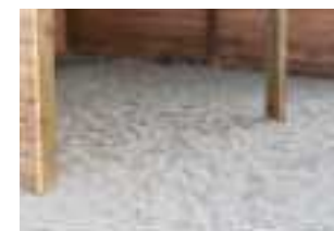
Sand or fine stone is used for the top layer, about 3/4" to 1 3/4" deep or more.
